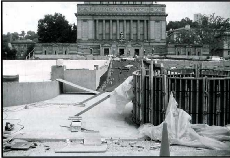
Construction progress of multi-level underground parking structure in front of Soldiers & Sailors Memorial. Landscaping will restore site to original sloped condition.
